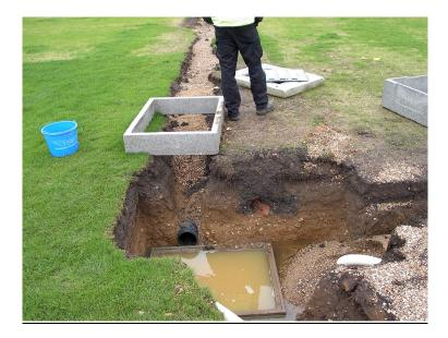
An example of new drainage installation. The ground might be contaminated with chemicals which could be leached off site to controlled waters.
